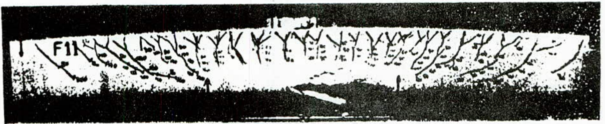
Fig. 11 Crack pattern in a plated beam
